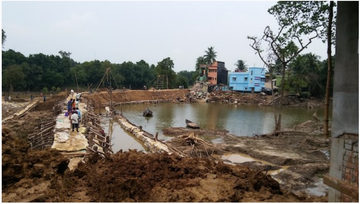
All that remains of the bund at Pratappur (Photo: Aditi Roy Ghatak)
